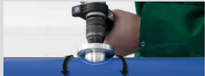
Removal of the oxygen barrier layer from the aquatherm blue pipe of
