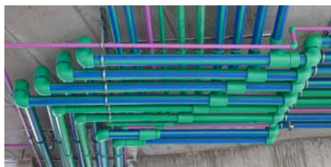
The connection of floor heating systems or the installation of radiator pipes up to the manifold can also be carried out with aquatherm blue pipe.
