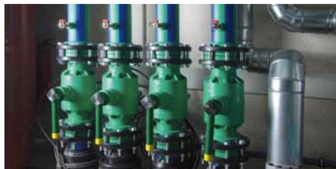
Risers and distribution piping for heating supply should be planned and installed with aquatherm blue pipe - faser composite pipes.
