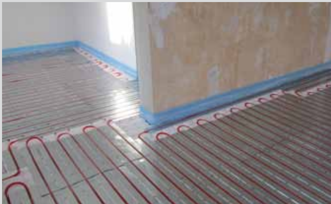
Completed heating system TS
