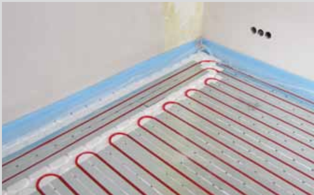
Completed heating system TS
