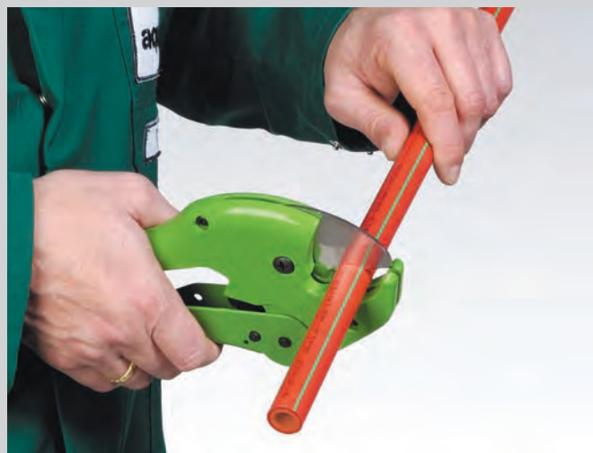
Cutting of the pipe
