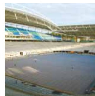
Undersoil pitch heating
