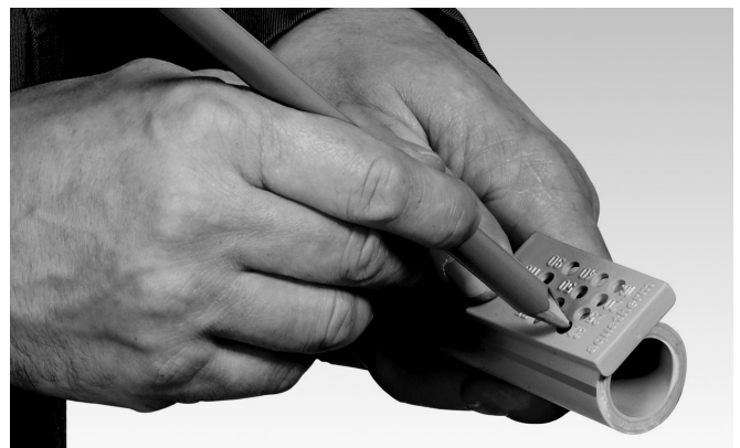
Marking of the welding depth
