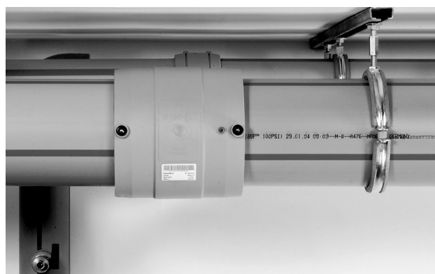
Push the second pipe - also peeled and cleaned - into the socket
