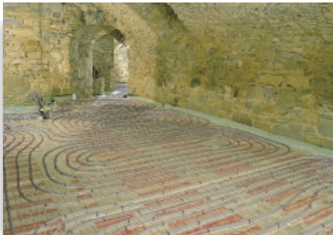
▲ Spiral-type placement in a movement zone
