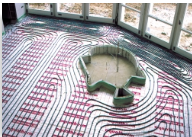
▲ Arrangement of different heating circuits
