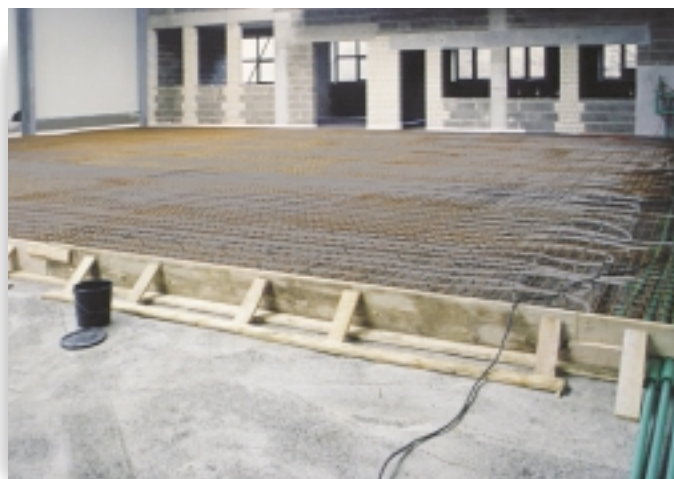
▲ Installation industrial floor heating
