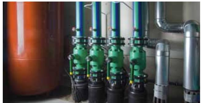
Risers and distribution piping for heating supply should be planned and installed with aquatherm blue pipe -faser composite pipes.
