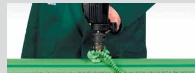
Drilling through the pipe wall
