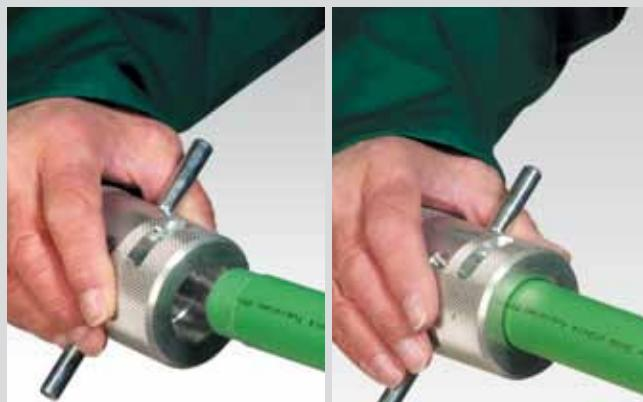
Peeling of the aluminium-PP-composite-layer respectively oxygen barrier layer (Necessary only for stabi-composite pipes and aquatherm blue pipe OT)
