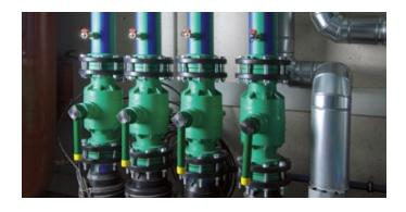
Risers and distribution piping for heating supply should be planned and installed with aquatherm blue pipe fibre composite pipes.
