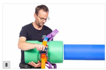
Final insertion of the pipe into the fitting must be done with an alignment tool.
