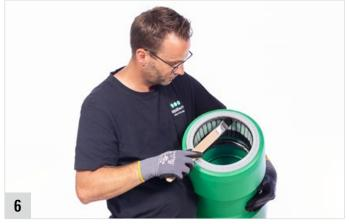
Apply lubricant also on the rubber gaskets of the push-fit fitting.
