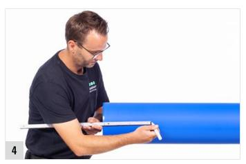
... and mark the insertion depth on the pipe.
