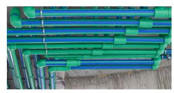
The connection of floor heating systems or the installation of radiator pipes up to the manifold can also be carried out with aquatherm blue pipe.
