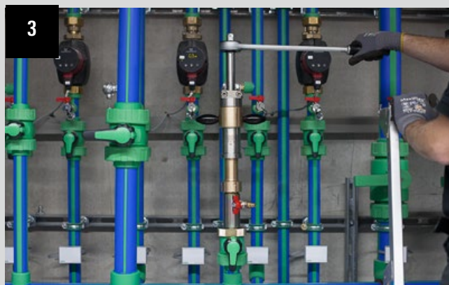
3. Start of the drilling process
